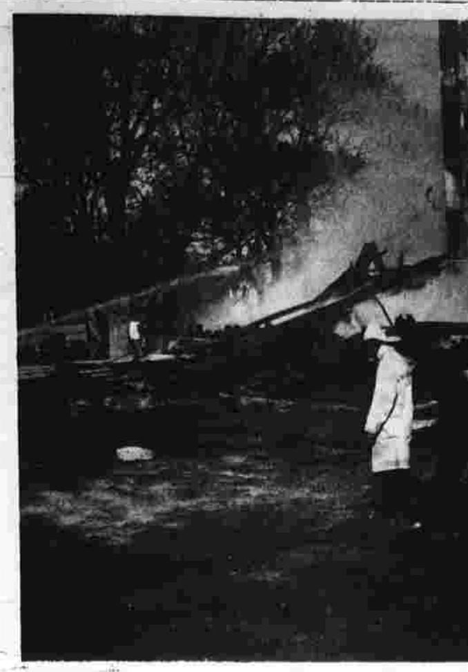
What's left of the Lebanon town building. (Other photo, details on Page 1)
